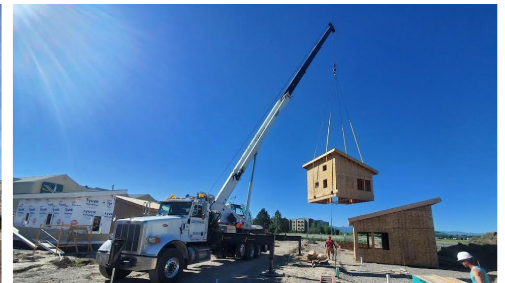
The tiny homes are placed on foundations using a crane.
